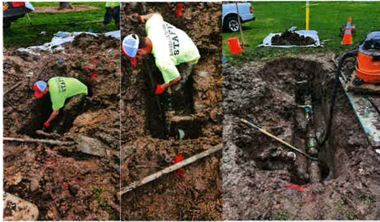
Six Inch Main Repair @ Freedom Park
