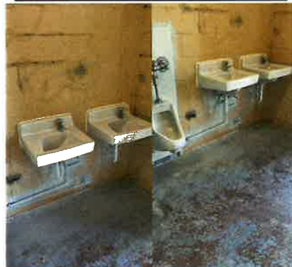
Brock Park Restroom Remodel
