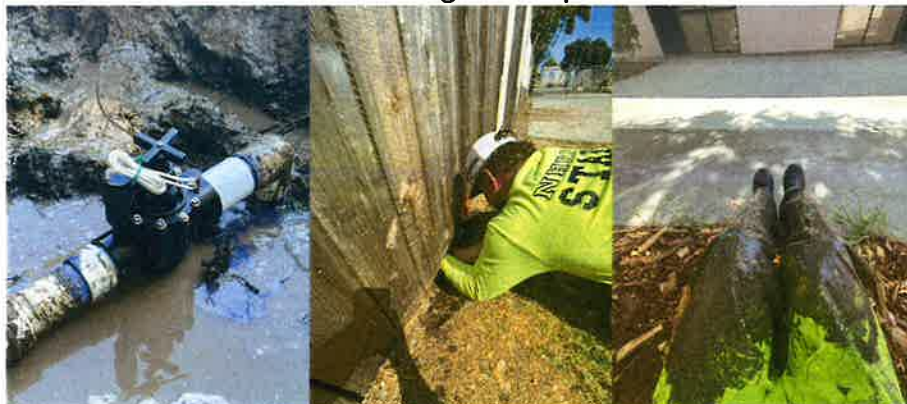
Various Irrigation Repairs
