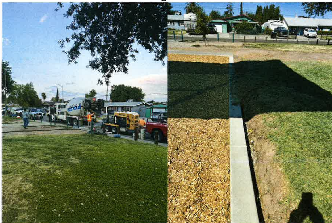
Concrete Work @ Karl Rosario Park
