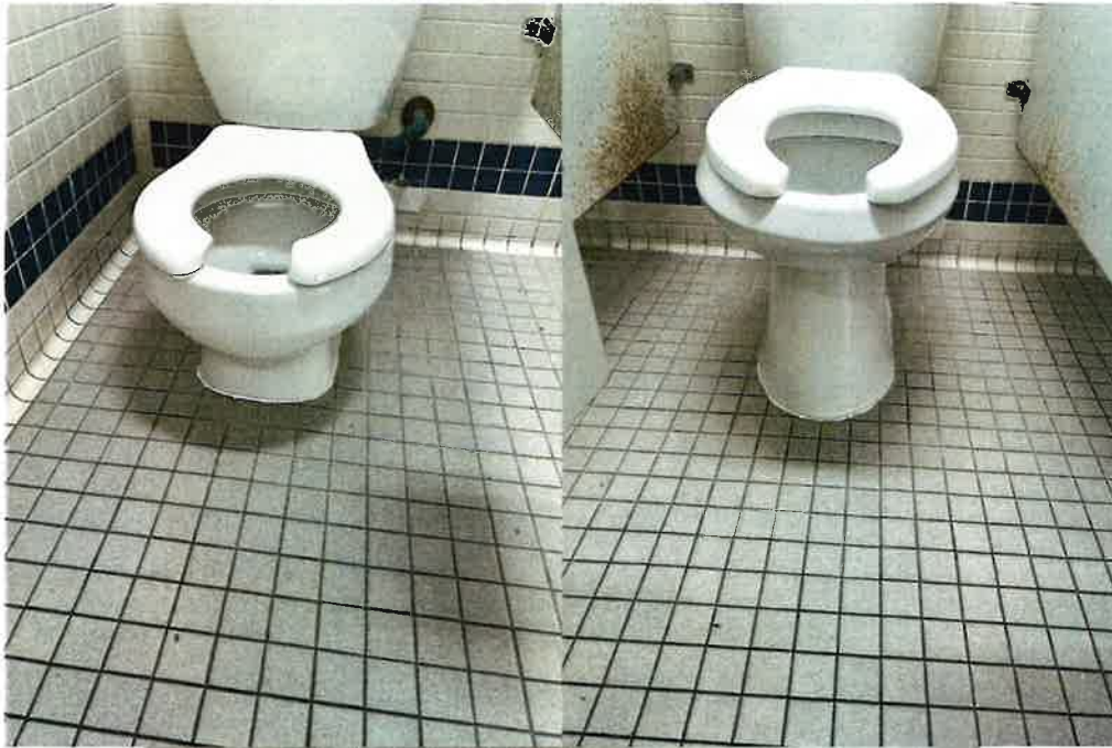
Repaired Toilets @ Something Extra Preschool
