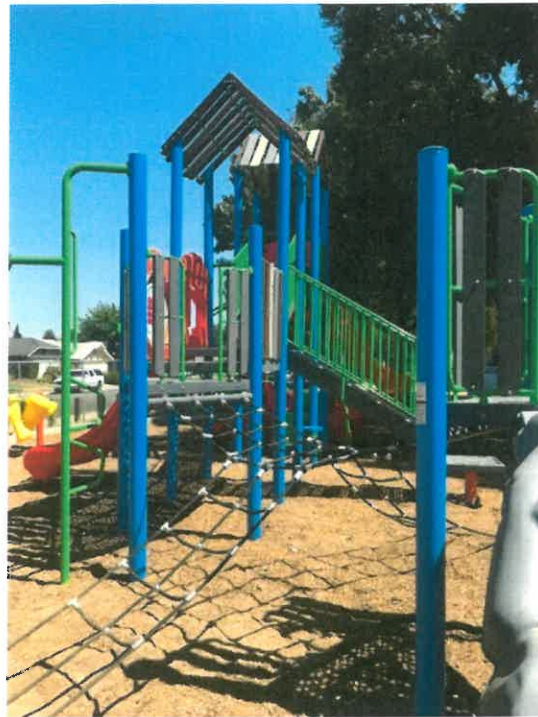
Ridgepoint (playground install complete)
